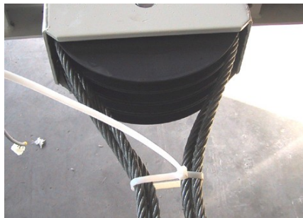
Figure 24: Temporarily bind the cables together
