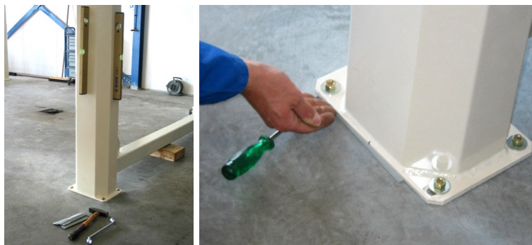
Figure 11: Vertical position of the columns
