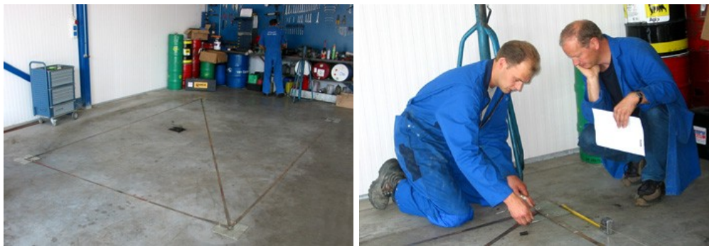
Figure 5: Determine the drilling points with the drilling jig
