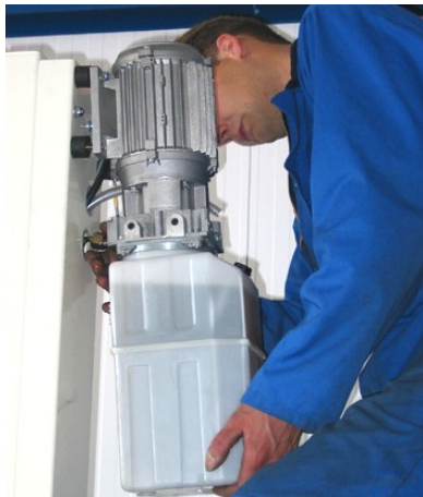
Figure 16: Install the hydraulic unit
