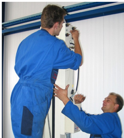
Figure 14: Installing the control box
